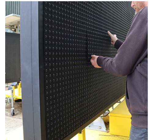
A VMS panel being replaced by one of our Engineers
