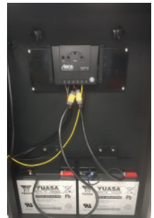
2 batteries and Solar Charge Controller
